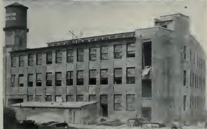
Upper, Starting Excavation, Jan. 8. Lower, Building Complete March 8.
